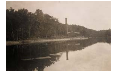
Figure 7 ~ Campbell's Pond with the pumping station in the distance.
