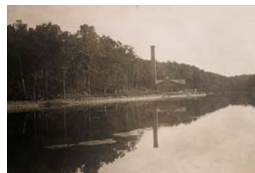
Figure 6 ~ Historic Pumping station for the City of Orange.
