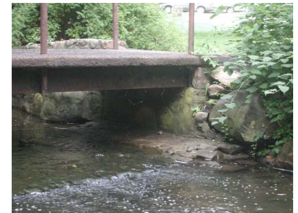
Figure 83 ~ Foot bridge at replaced from the original set on the abutments
