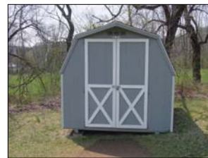
Figure 68 – Archery storage shed.
