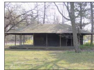
Figure 67 – Abandoned structure. Appears to have been a concession stand.
