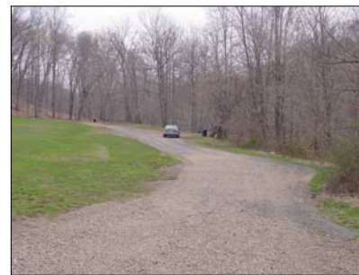
Figure 53 – Access road is gravel after the paved connection to Brookside Drive.
