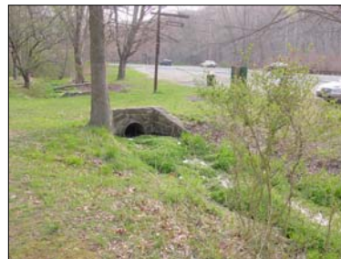
Figure 51 – Parking and drainage with culvert and headwall at Elmdale Picnic Area.
