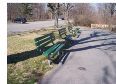
Figure 88 ~ Viewing area at Bramhall Terrace showing benches in need of replacement.
