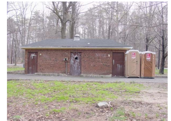
Figure 82 ~ Tulip Springs picnic area restroom building with portable toilets .
