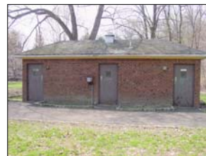
Figure 66 – Non-functioning restrooms. Port-a-johns are provided.
