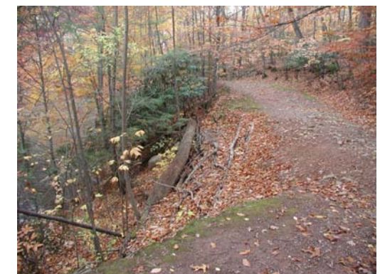
Figure 79 ~ Erosion occurring on steep slope with little ground cover adjacent to River Trail.
