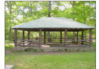
Figure 72 – Mayapple Hill shelter showing massing similar to original design with different material.
