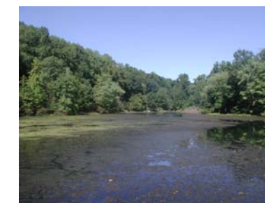
Figure 50 – Diamond Mill Pond Dam
