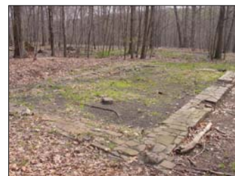
Figure 56 – Picnic shelter remnants from original shelter.
