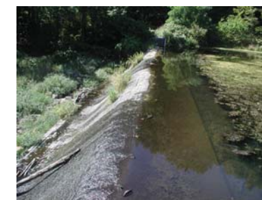
Figure 49 – Diamond Mill Pond Dam
