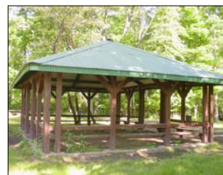
Figure 71 – Original shade structure with new roof. Internal bench is missing.
